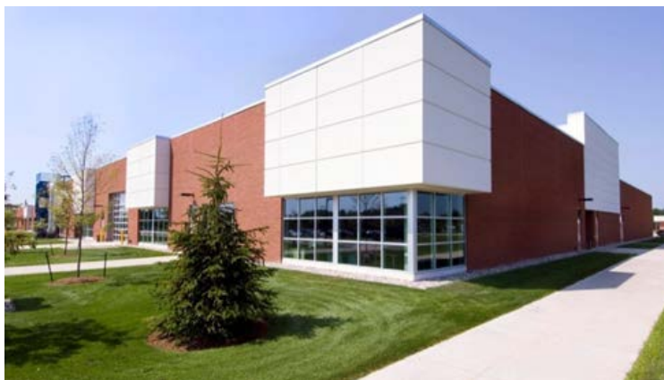
Delta College Technical Trades & Manufacturing Complex
