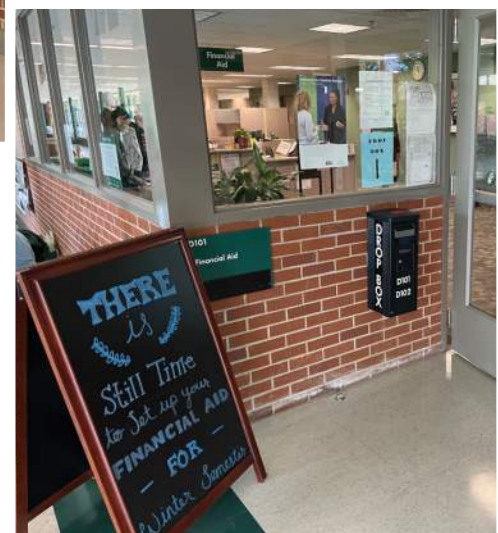
Temporary A-frame blocks room identification sign. Current location of room identifier is too low.
